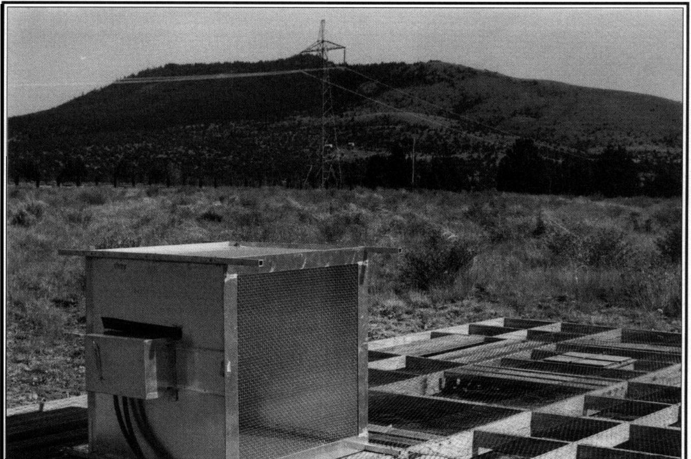
Figure 6.5. Long-term measurements were made of the electrical environment of the DC Intertie line near Grizzly Mt. in Central Oregon. The box-like device is a space charge cage used to measure air ions and charged aerosols at distances out to 610 m (2000 ft) from the line. A 1 m (3.3 ft) square Wilson plate used to measure the DC electric field is located in the wood framework to the right of the cage. Source: Chartier et al. (1989).
