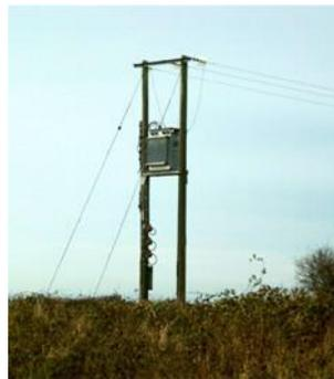
The fields from these transformers fall off very rapidly and are usually negligible further than 3 metres away - the fields from the overhead wires are usually more concerning, and the 11 kV wires should not pass within 20 metres of the house.
